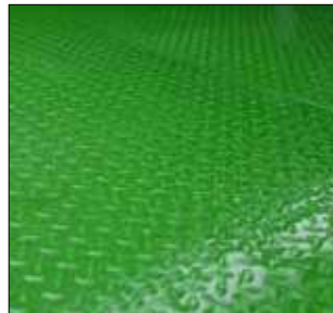
FLOOR - chequered steel plate with drainage openings
